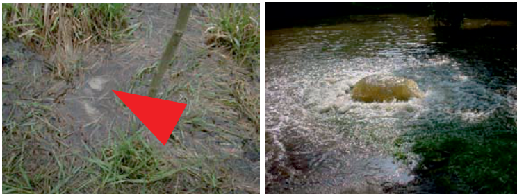
These photos show examples of water discharge points on the landside of a dyke Photo credits: THW Emden
